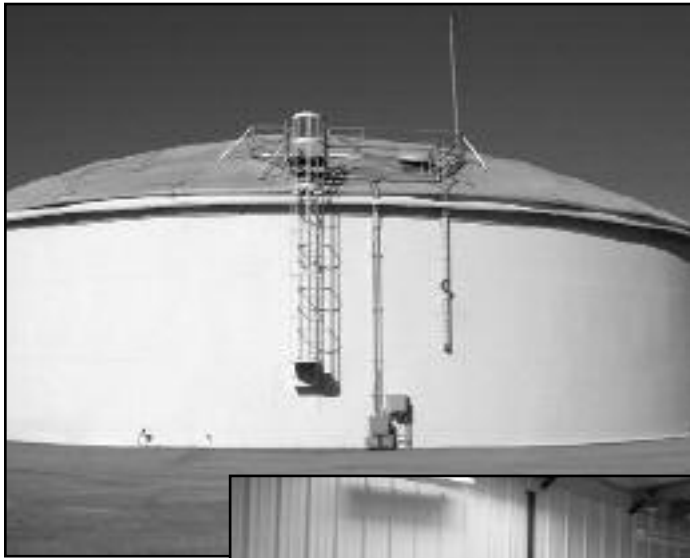
The new 2 million gallon water tank northeast of Aten and Cross roads.
