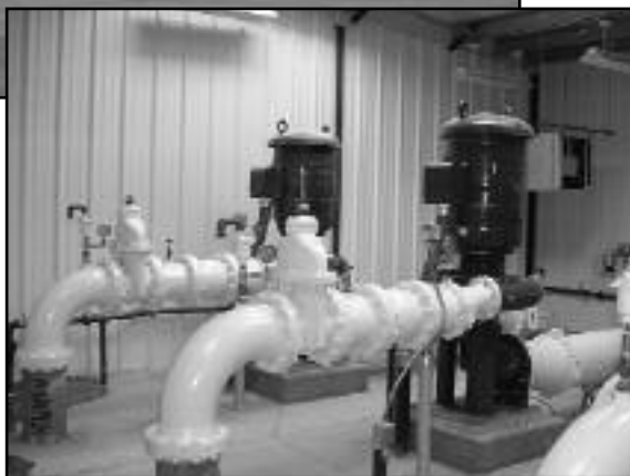
One of the 2500-gallon-per-minute pumps at the new 2 million gallon water tank serving Imperial's rapidly growing southeast section.
