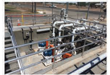
B street pump station completed in 2016
