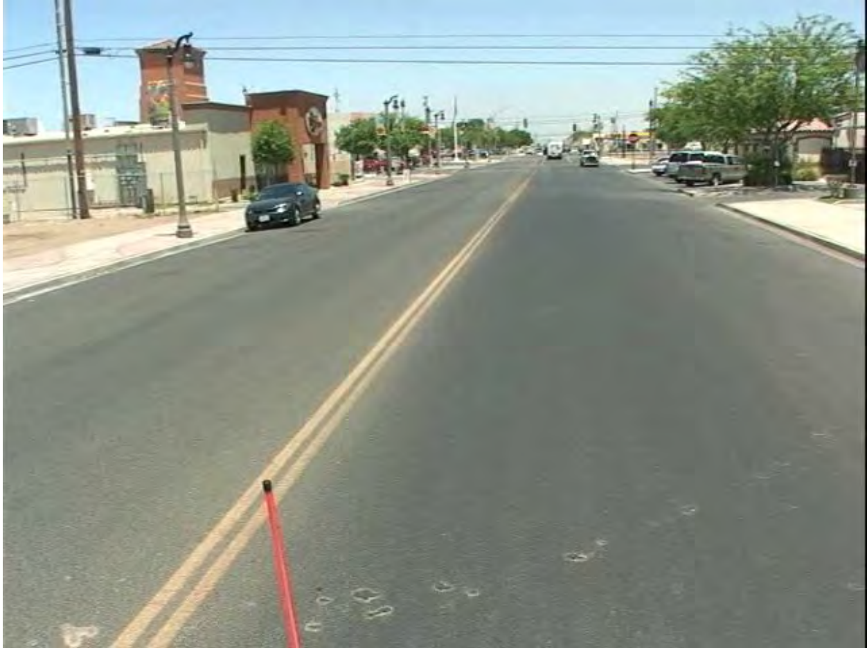
Barioni Blvd, PCI = 92 and the Surface is Distress Free, Smooth and Ready to Provide Years of Good Service
